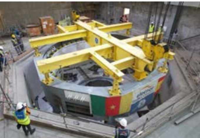
Nachtigal's last stator installation's pictures
